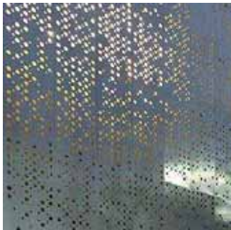
SF01 - SOFFIT PERFORATED ALUMINUM PANEL - SILVER COLOUR - BACKLIT FEATURE - ANODIZED FINISH
