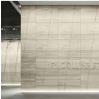
ST01 - SANDSTONE WALL CLADDING - COLOUR WHITE RANGE FINISH SMOOTH
