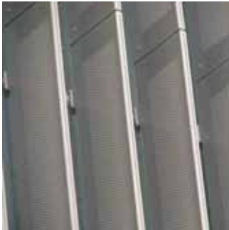
PF01 - PERFORATED ALUMINUM VERTICAL LOUVRES - COLOUR SILVER - ANODIZED FINISH
