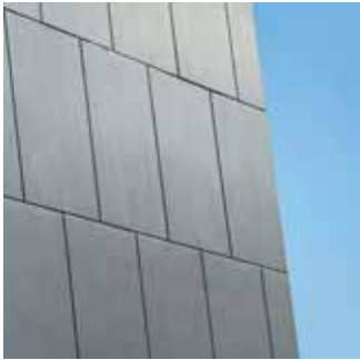
CP01 - PRECAST CONCRETE PANEL - COLOUR CHARCOAL/BLACK - APPLIED FINISH
